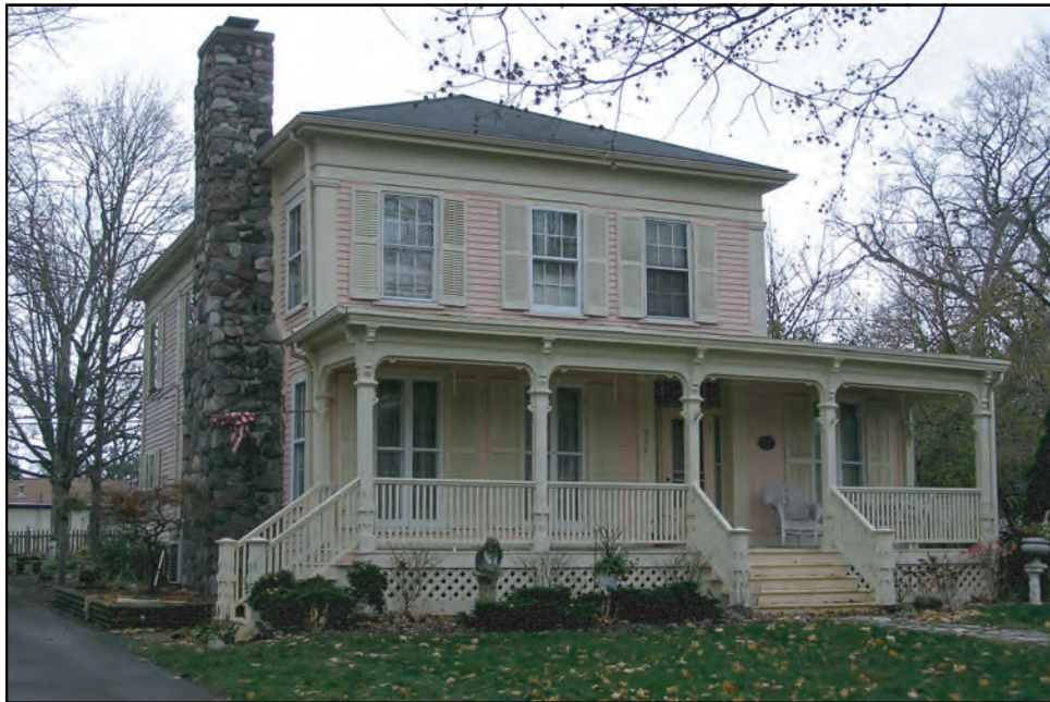
Figure 3.2.1-8. Andrew Grover Residence, 233 West St. Clair Street, North and East Elevations
